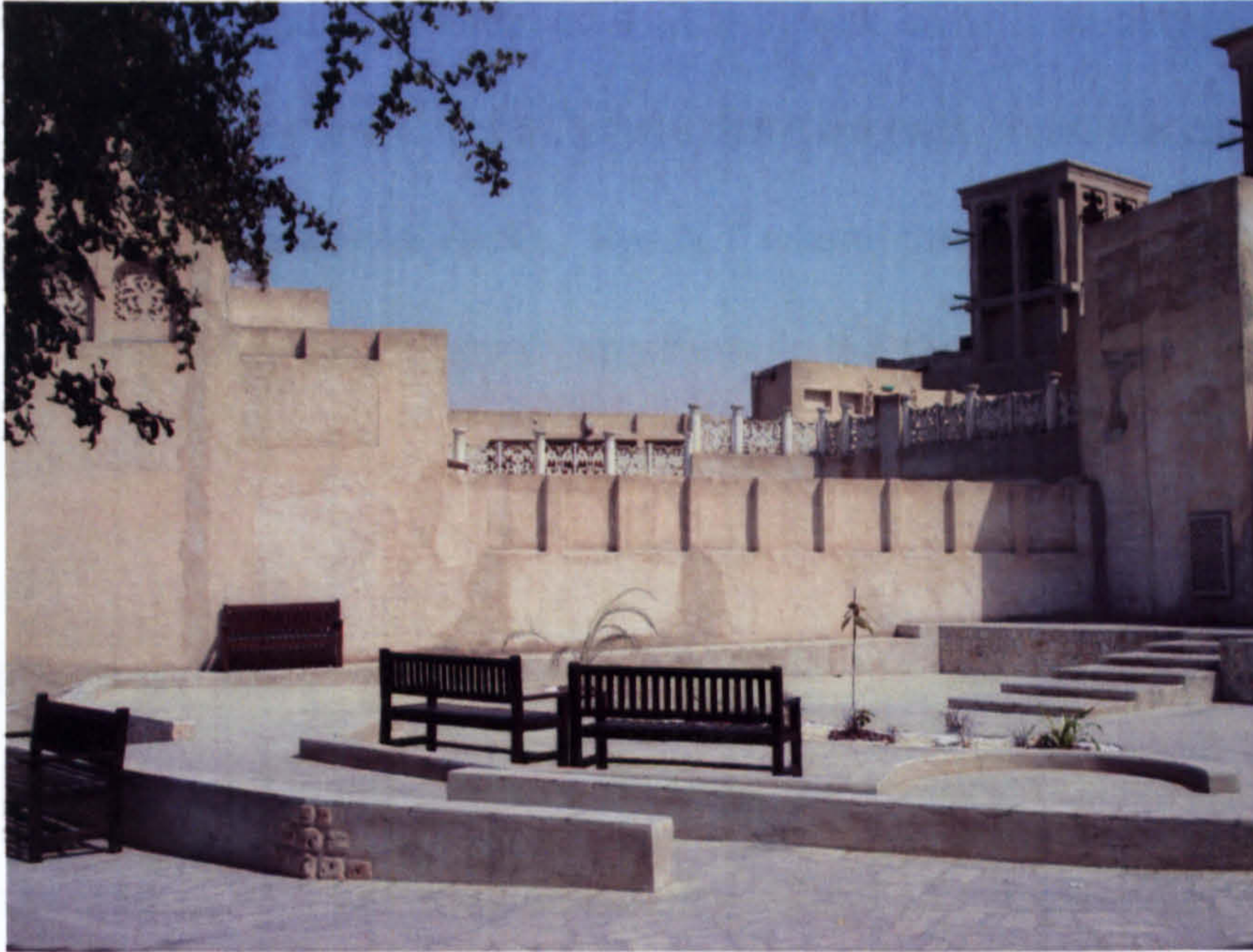
Figure 13. Symbols of old Majless in Albastkiya destrict in Dubai – source: photo is taken by the author2006
