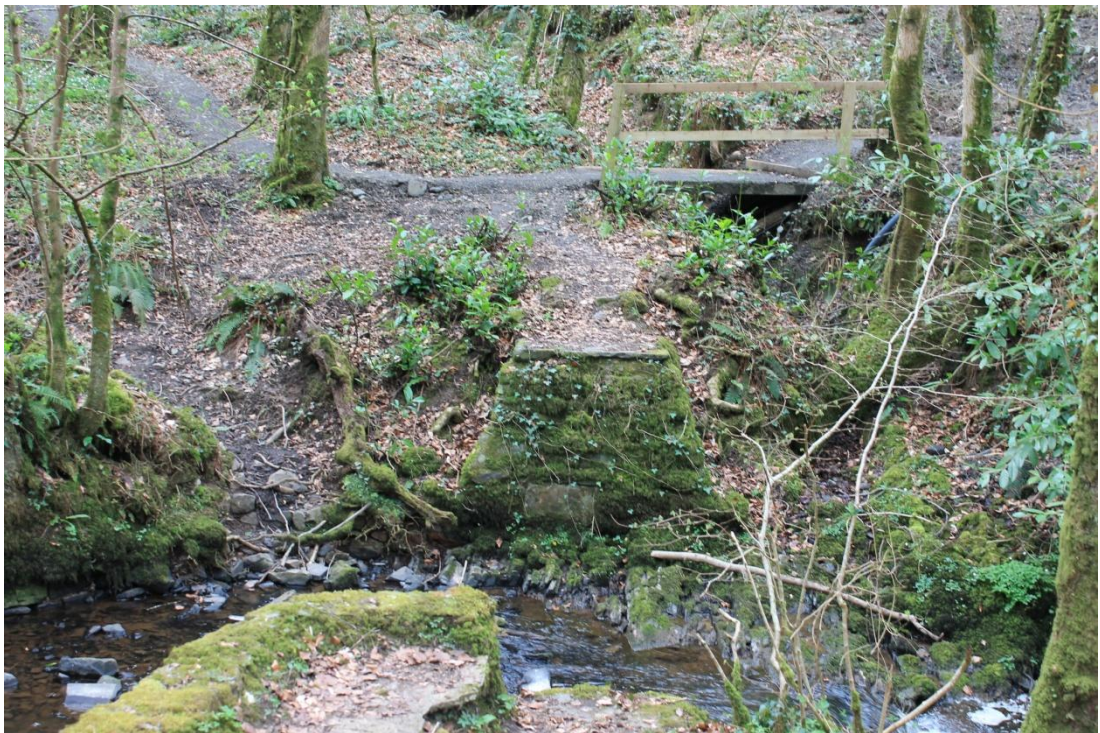
Damaged Footbridge at Pont Felin-gât
