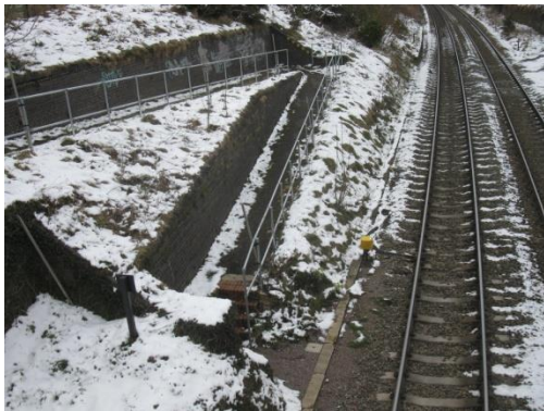
Figure 10: Left: The 'up' line (i.e. towards Hereford) at Llanfihangel, looking down from the bridge (see above), showing the zigzag path up to road level. The remains of the platform are bottom left.
