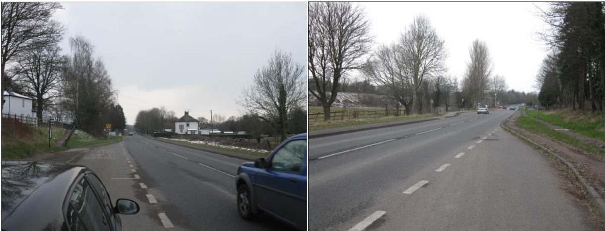
FIGURES 7 & 8: Above: The A465 through Pandy facing west (to Abergavenny) on the left, and facing east (to Hereford) on the right. This road, built in the 1960s, replaced the twisting old road through Pandy and made it difficult to keep a sense of a cohesive community. The effects of this road were foretold by Morgan Rosser in Border Country who saw its inevitability even in the 1930s, and in The Fight for Manod Matthew Price and his wife Susan revisit Glynmawr at the end of the novel and notice the changes it has brought: 'The new straight road for the lorries was thirty yards back ... Farther into the village, the straight line of the new motor road had changed the shape of the valley and its settlement'. pp. 203, 204 of The Fight for Manod (London: The Hogarth Press, 1988 edition of novel first published in 1979).
