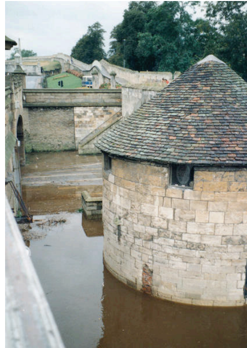
Frequent flooding and the tower's position has resulted in damp in the ground floor stonework
