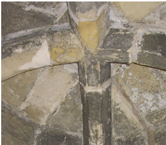
The internal stonework is subject to decay
