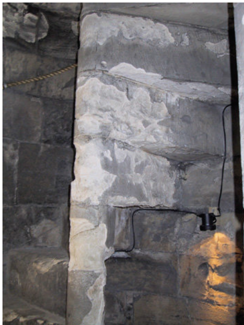
Severe decay of the spiral staircase in the Tower may cause structural concerns in the future
