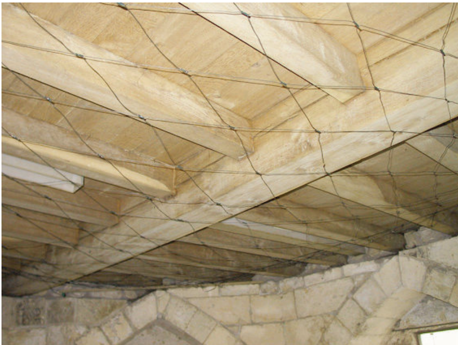
The main beam supporting the first floor flags is cracked along its length
