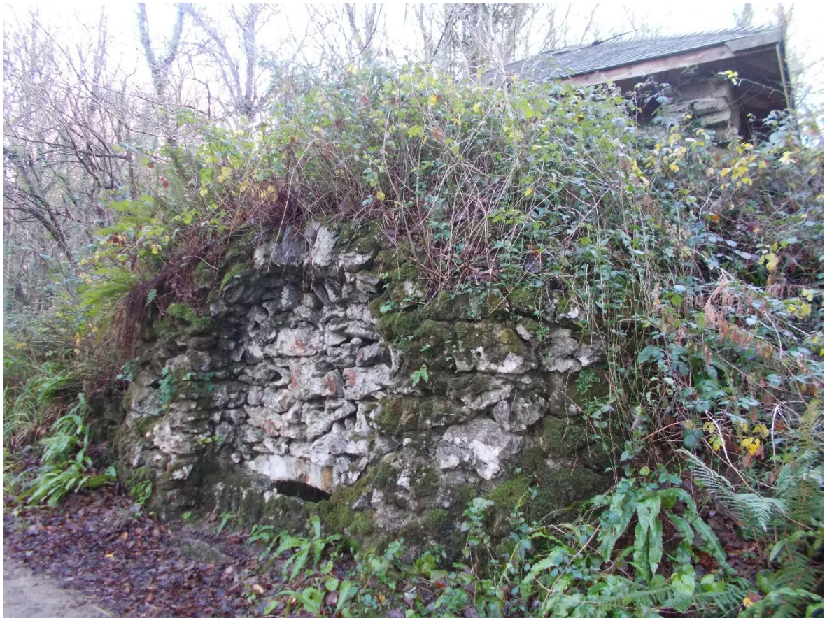
Figure 82 - Remains of the Stackpole Court ice house in rustic limestone, © Daniel Evans 2016
