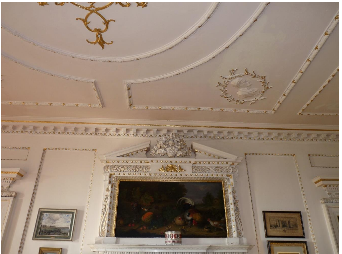
Figure 126 - Misalignment between chimney piece overmantel and centre of ceiling decoration in the White and Gold drawing room, indicating two phases of work, © Daniel Evans 2015
