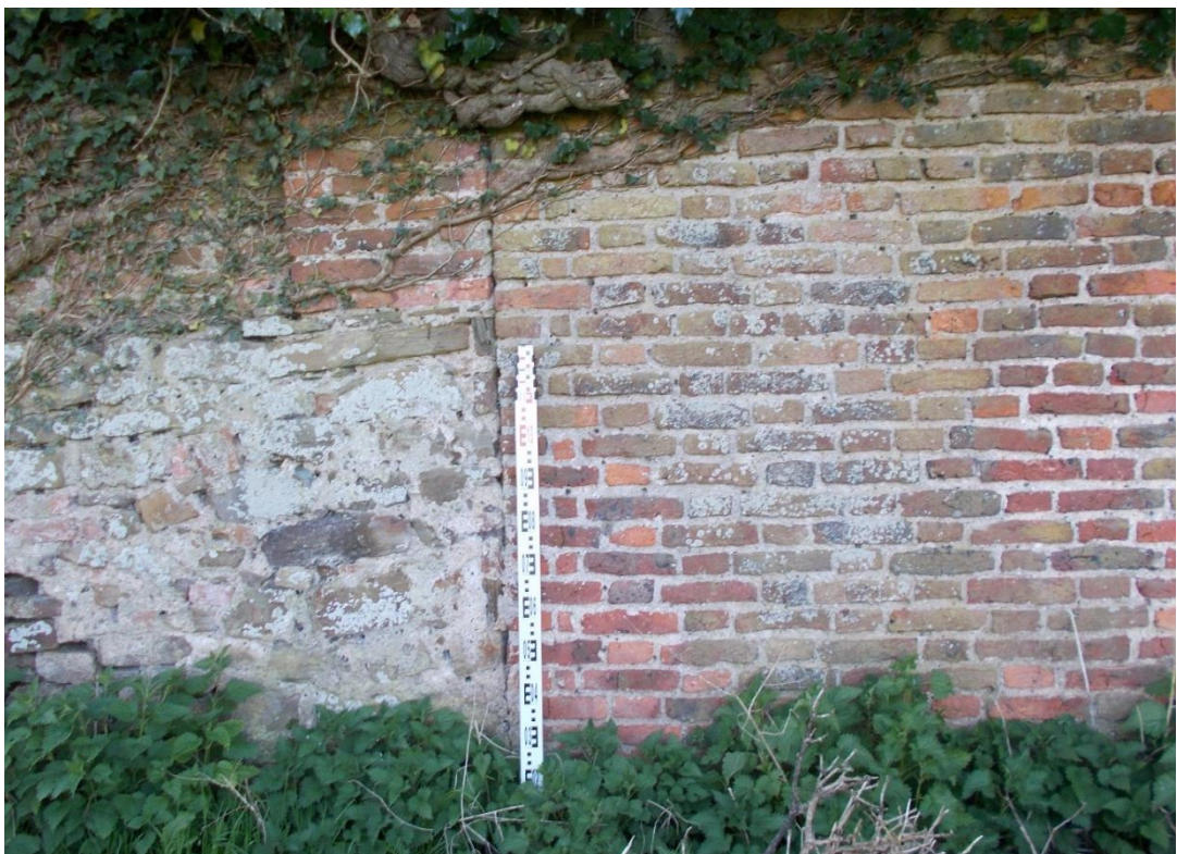
Figure 11 – Abutment of NE summerhouse with the stone footings to the brick wall with arched openings, © Daniel Evans 2018
