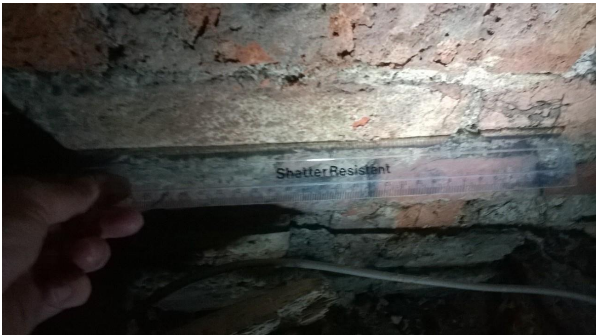
Figure 76 - Brickwork inside the parapet of the orangery, © Daniel Evans 2015
