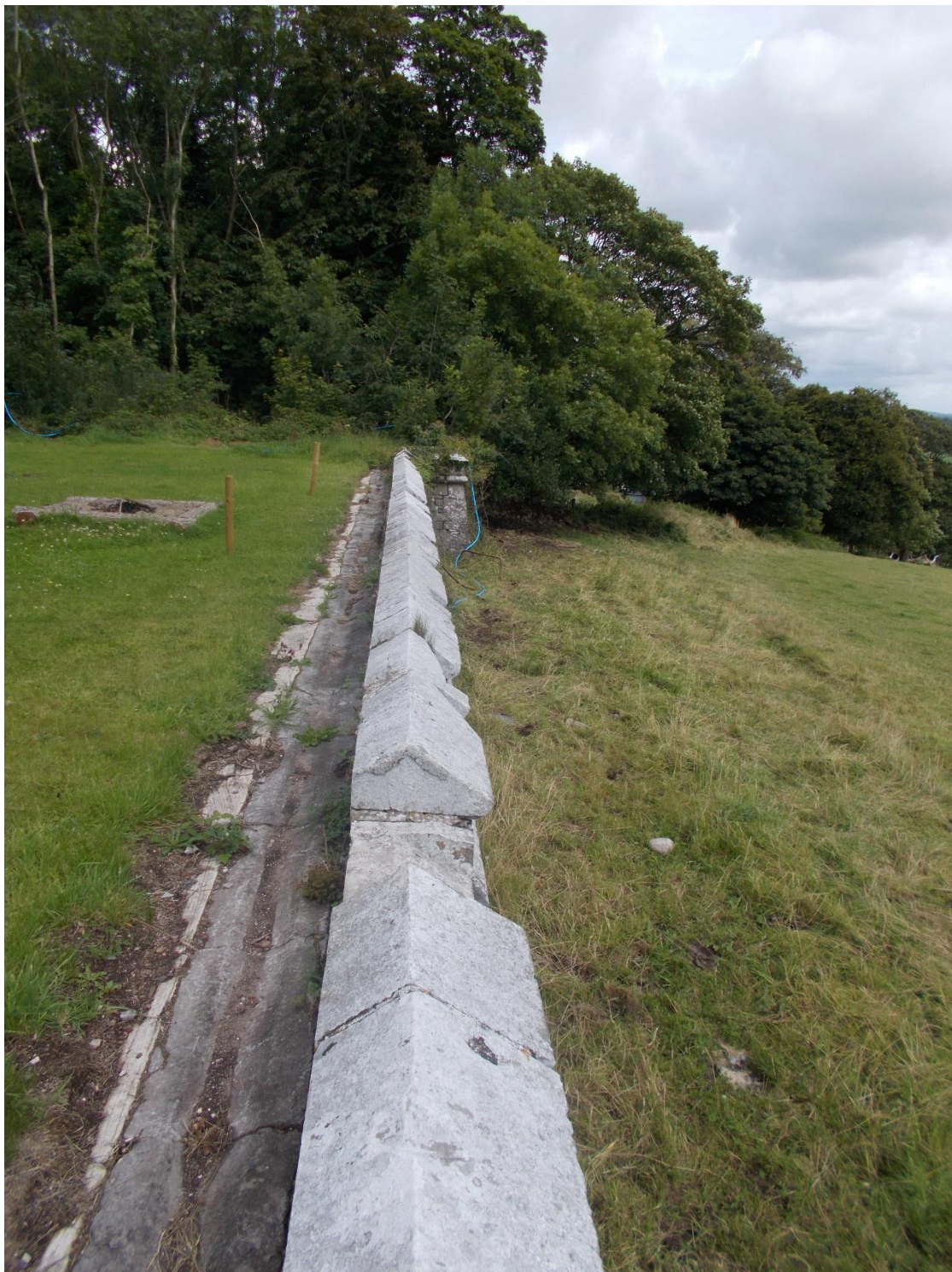
Figure 39 – Castellated terrace looking NE © Daniel Evans 2018
