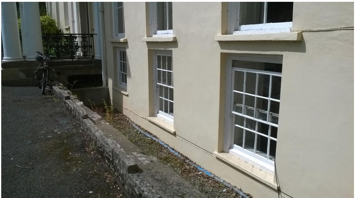
Figure 57 – Raised ground level and lightwell at the E entrance front, © Daniel Evans 2015
