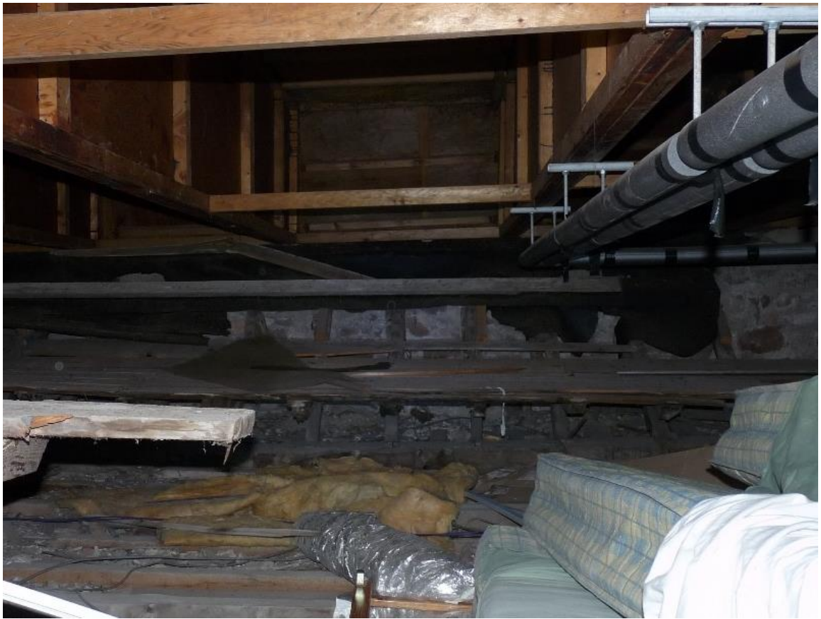
Figure 75 – Stonework face of the inside of the parapet at Orierton, © Daniel Evans 2015
