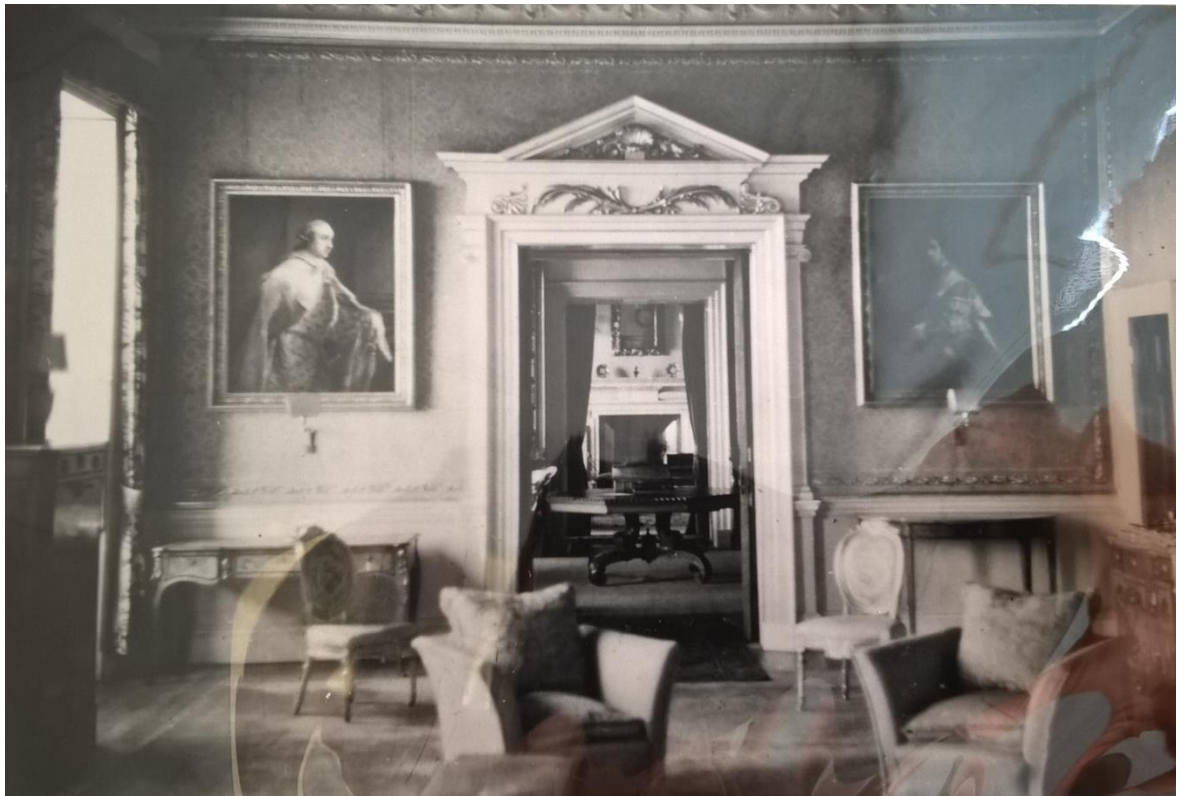
Figure 98 - Interior of Stackpole Court showing enfilade arrangement (RCAHMW BB72/3934) From the collections of the National Monuments Record of Wales: © Copyright: NMR Site Files
