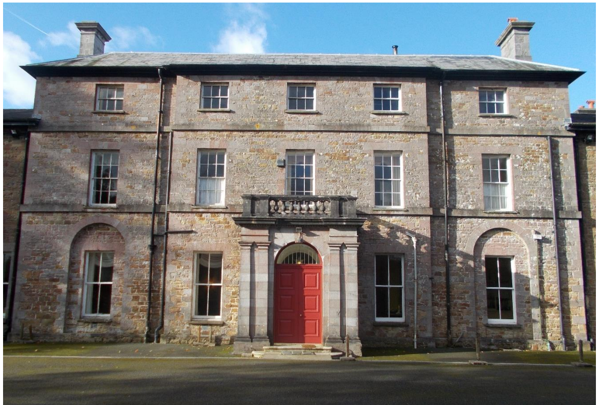
Figure 139 – Entrance front of Cresselly House dressed stone details similar to those at Brownslade, later porch of 1869 © Daniel Evans 2017
