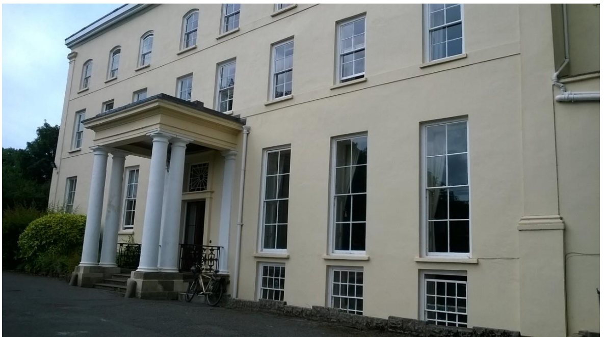
Figure 62 - Orielton E entrance front, with remaining portico, © Daniel Evans 2015
