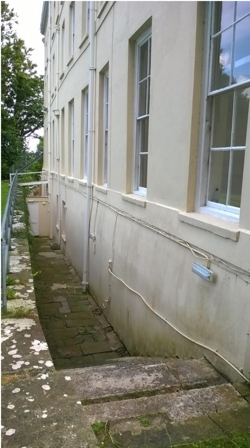
Figure 58 – Raised lawn and lightwell at W front of Orielton House © Daniel Evans 2015
