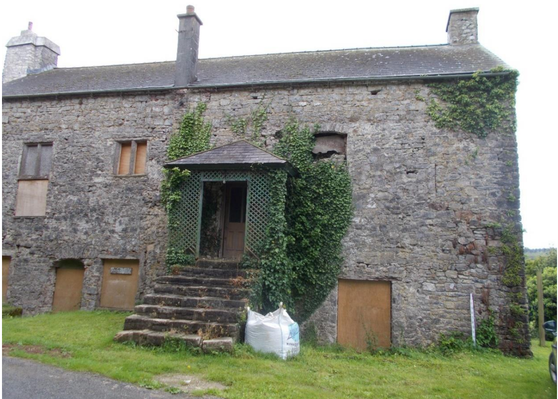
Figure 23 – North elevation of Coedcanlas house with the porch added c.1810 © Daniel Evans 2018
