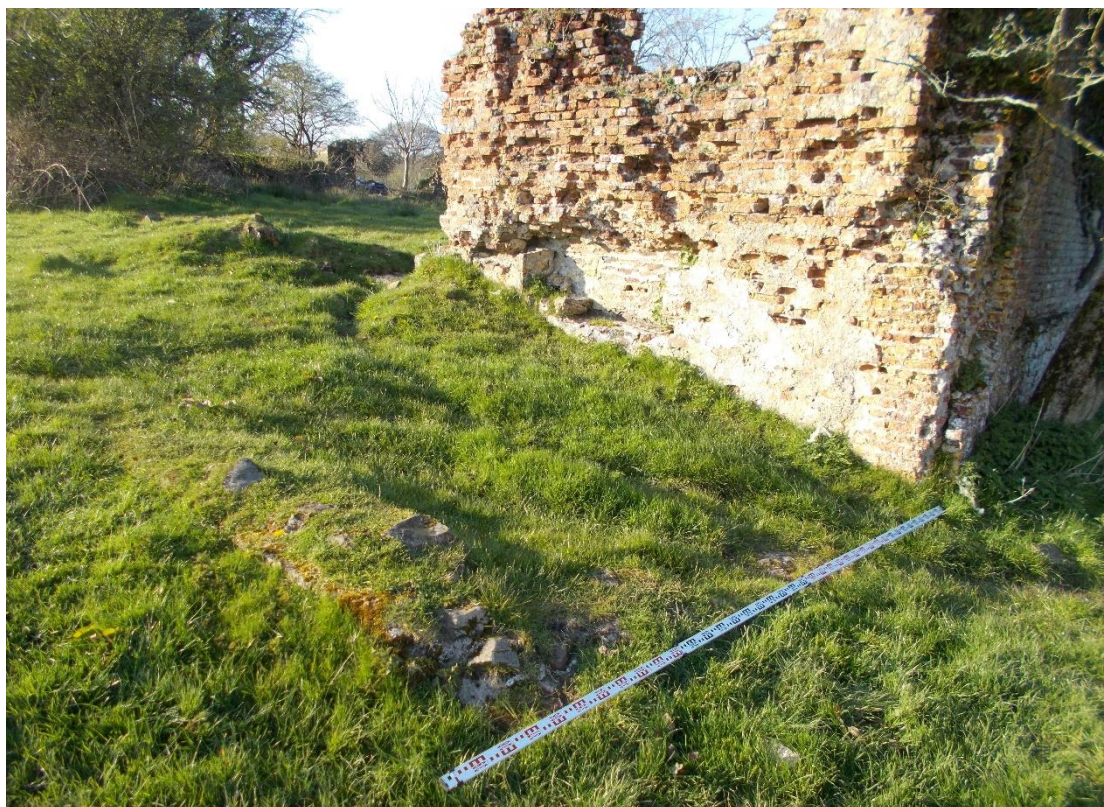
Figure 15 – Tumbled flank wall to SW summer house, with masonry footings as earthworks, © Daniel Evans 2017
