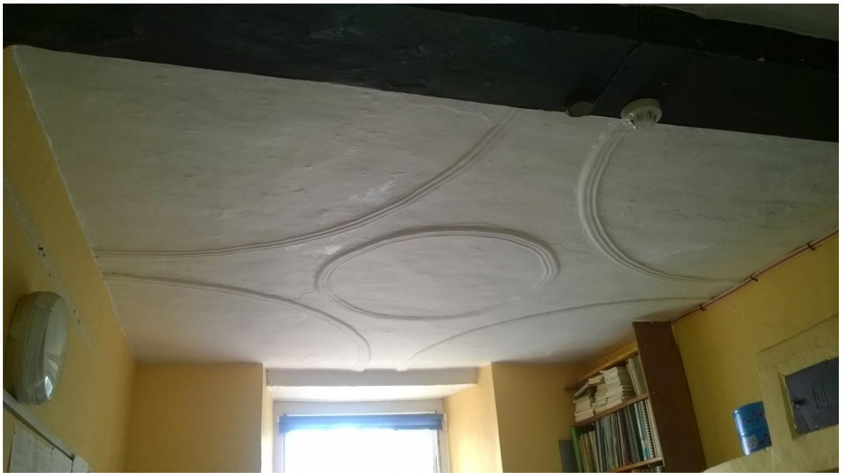
Figure 61 – C17 plaster ceiling in the basement at Orielton, c.f. Plas y Wern Ceredigion, © Daniel Evans 2015
