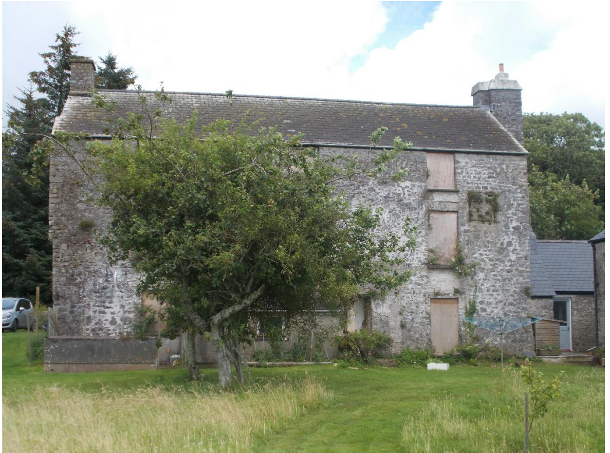
Figure 22 – South elevation of Coedcanlas house remodelled c.1810, © Daniel Evans 2018
