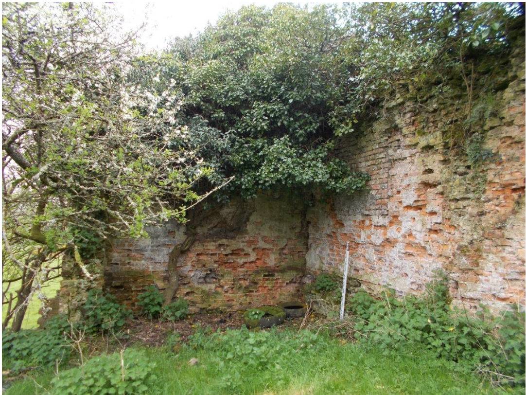
Figure 10 - Possible summer house at NE corner, Landshipping gardens, © Daniel Evans 2018
