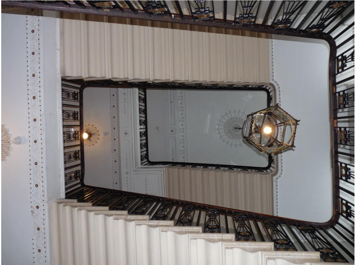
Figure 65 - Greek Revival cantilevered stone stairs at Orielton, © Daniel Evans 2015
