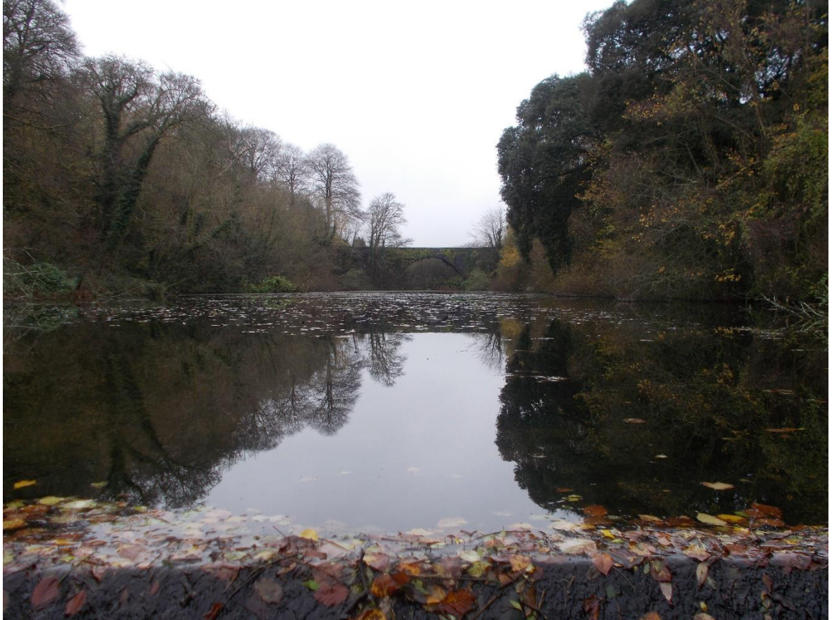
Figure 85 - View from the hidden bridge to the single arch bridge en-route to the Grotto, © Daniel Evans 2017
