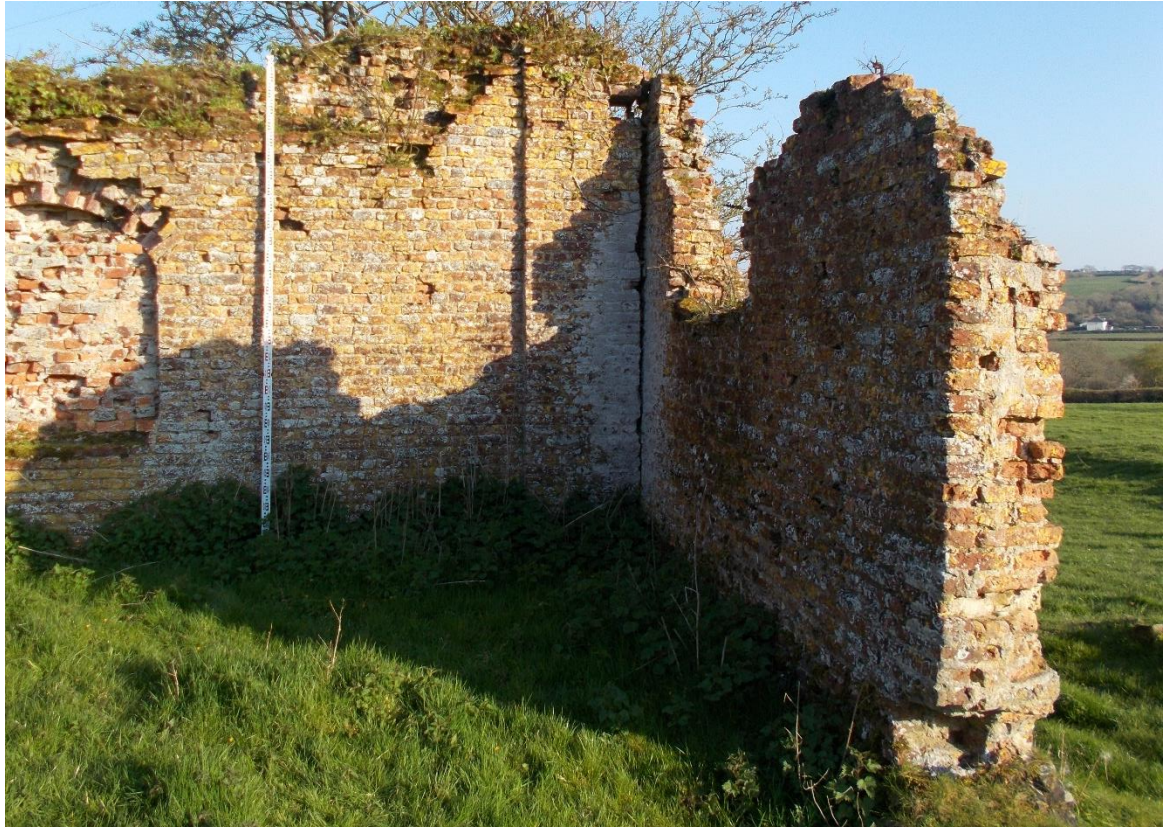
Figure 12 – Abutment of SW summerhouse with the wall containing arched openings, © Daniel Evans 2018
