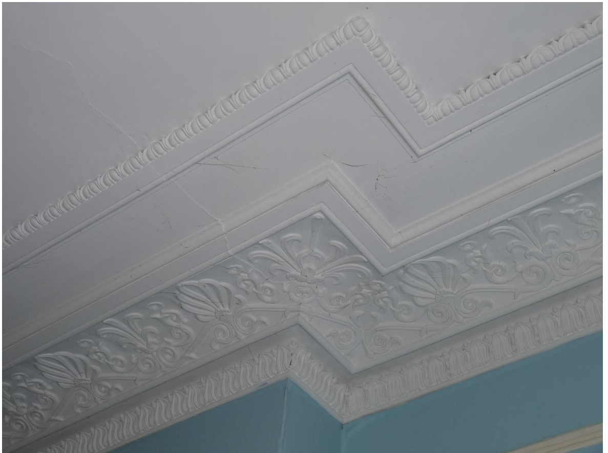
Figure 71 - Orielton dining room cornice, © Daniel Evans 2015
