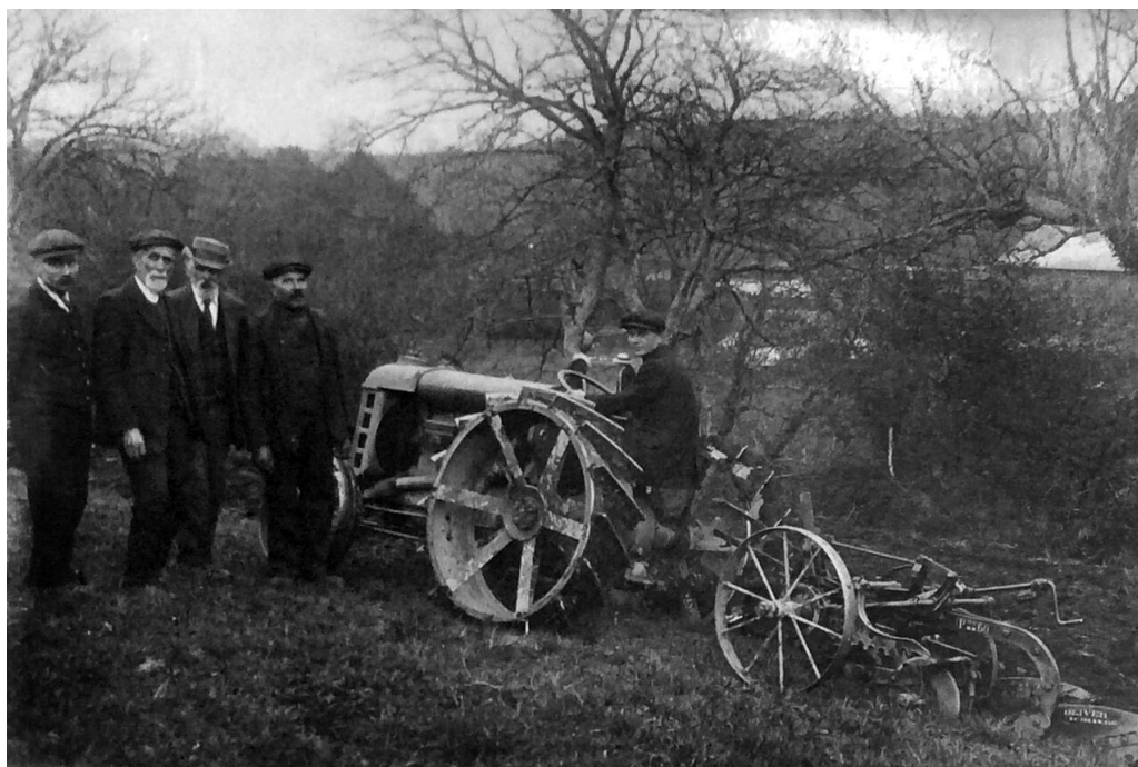
Figure 24. Ploughing the field above Scotchwells to make allotments for the Dig for Victory Campaign during the First World War
