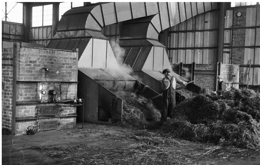
Figure 8. Grass-drying plant at Penrhos Aerodrome, Pwllheli, 1948
