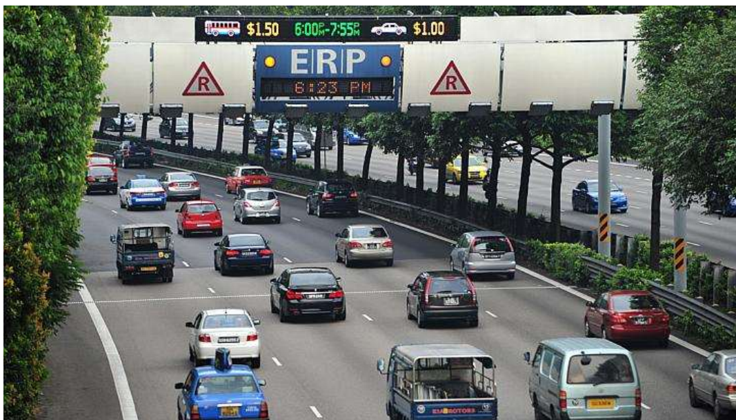
Figure 2.15: An Electronic Road Pricing (ERP) Gantry (source: All Singapore stuff)
