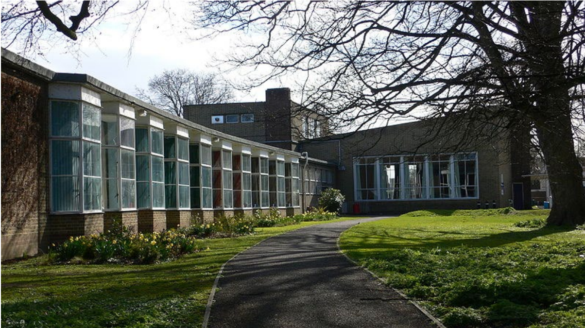
Impington Village College
