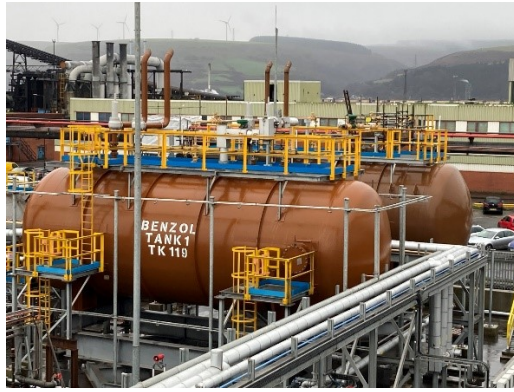
Figure 3: Completed case study project Benzole storage tank installation.
