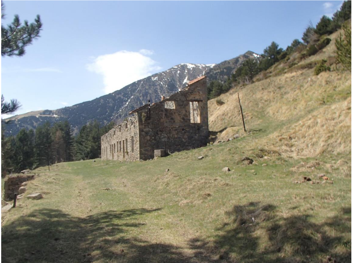
Figure 4.3 The sleeping quarters, mine de Batère, Corsavy (source: S. Jenkins Carter).
