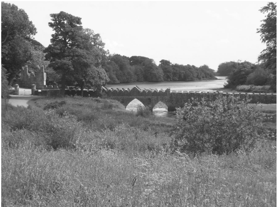
Tintern de Voto Bridge - Looking South towards Bannow Bay
