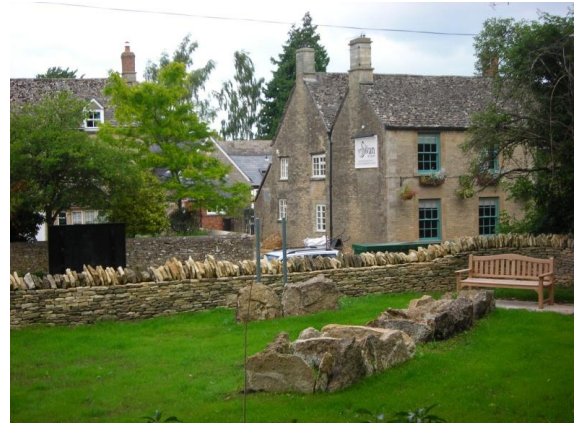
Fig. 69. The excavated Ascott stone cists, currently located near Ascott-under-Wychwood's Church. 335
