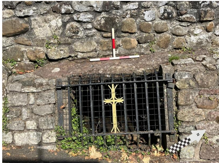
Figure 6: The grille and basin evidence erosion; rust, climbing plants and silt depicted. The differentiated masonry of the well-setting (bottom) and well-house (top) may indicate phased construction. Author, 19/07/2024, 11:02.
