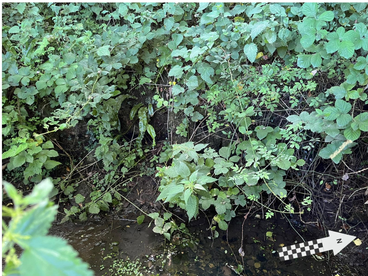
Figure 11: Larger sections of masonry were visible behind plant growth from the west (centre), however, erosion and overgrowth were significant. Author, 19/07/2024, 16:36.
