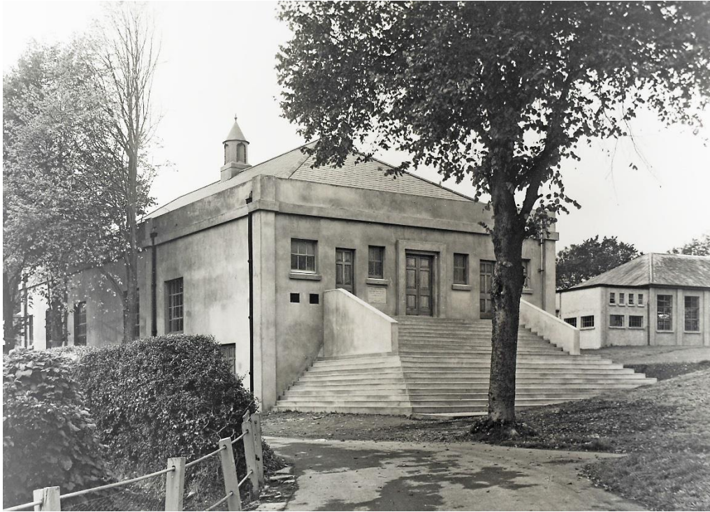
Exterior of Broadcasting Hall c. 1938
