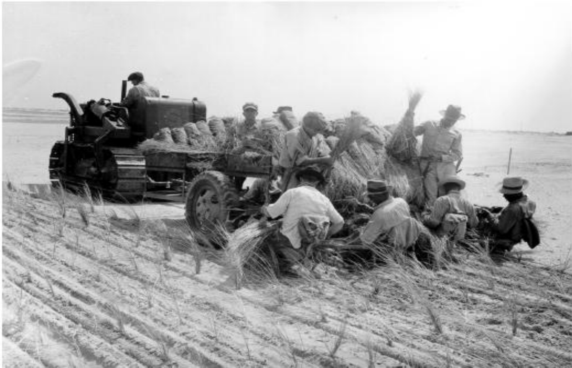
Figure I-3-12. Workers planting grass on a beach restoration project. The date and location of this image were not recorded, but the scene is likely the Outer Banks. Many dune and beach restoration efforts, sponsored by the National Park Service and other agencies during the late 1930s, also served as work relief efforts for a nation trying to recover from the Great Depression. Photograph from the Beach Erosion Board Archives
