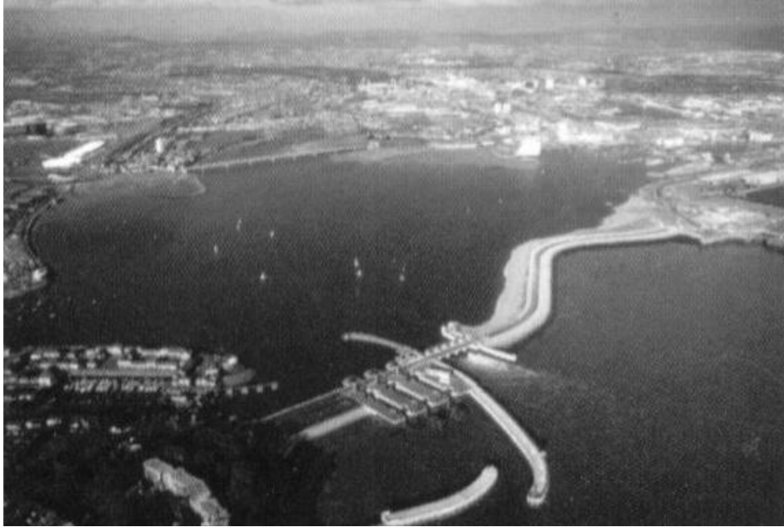
Figure 6: Cardiff Bay Barrage (Reproduced by kind permission of Balfour Beatty)
